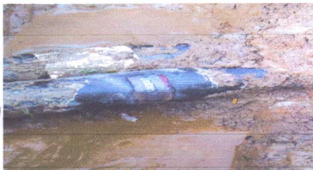
REPAIR WORK DONE BY NAOC REPAIR TEAM
