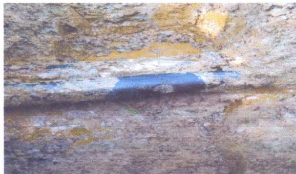
SPILL POINT AFTER EXCAVATION
